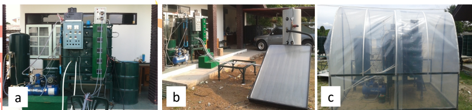
Figure 2. Three biogas production systems a) 1,000 L biogas production system without solar heating b) Solar collector connected to 1,000 L biogas digester system and c) Solar greenhouse covering the entire 1,000 L biogas digester system.
